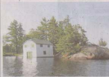
The existing boathouse on Wilcox Island. TAYLOR HANNAH ARCHITECT
